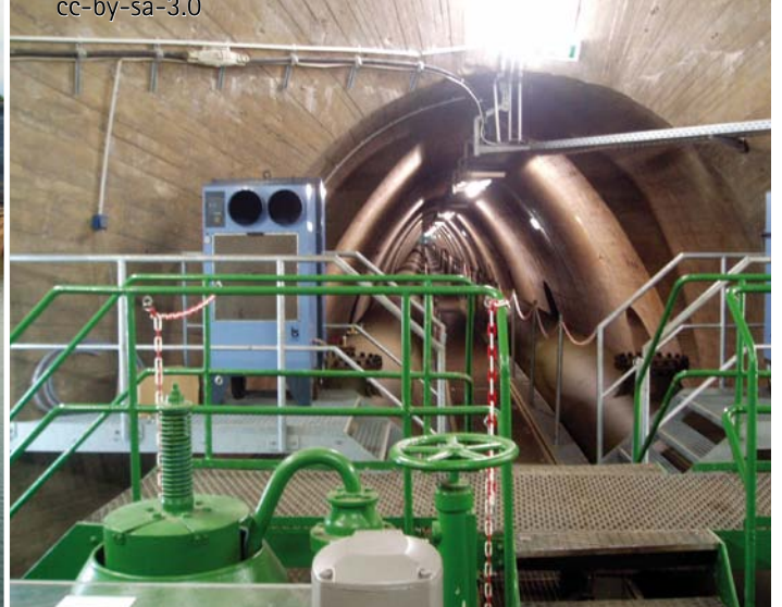
© Grundablassstollen Wahnbachtalsperre by Sebastian Appel | cc-by-sa-3.0
